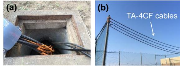
Fig. 4. Photographs of the installed TA-4CF cables at (a) the underground duct area and (b) the aerial area.
