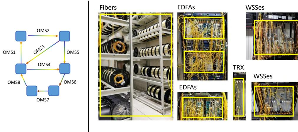
Fig. 1: The network topology (left) and a set of photos of the network equipment (right).
